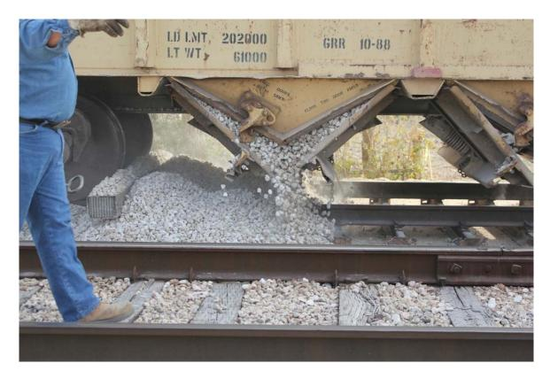
Over 3 million tons of Texas Crushed Stone's crushed limestone has been used for railroad ballast. Railroad ballast is typically graded from 1  $\frac{3}{4}$ " or 1  $\frac{1}{4}$ " to  $\frac{1}{2}$ ". Ballast is open graded and washed over a screen as part of the production process.
